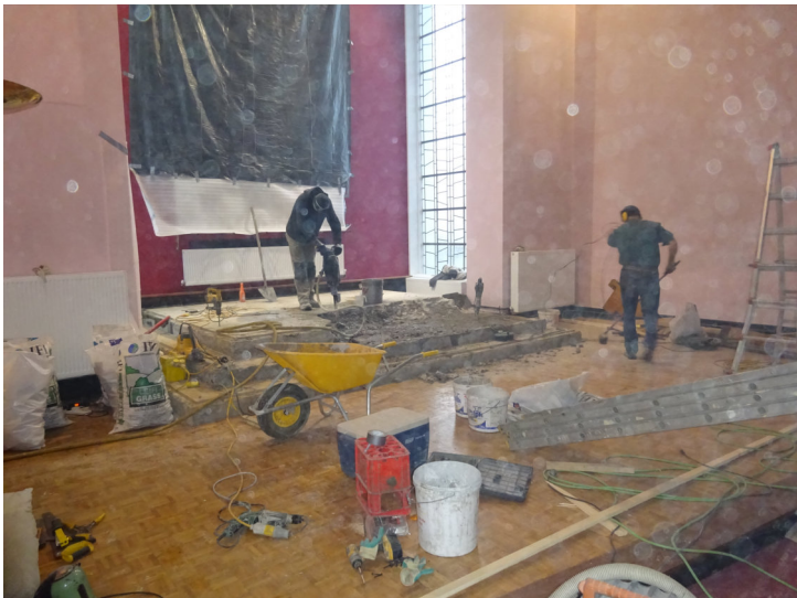
Workmen jackhammering out the concrete steps
